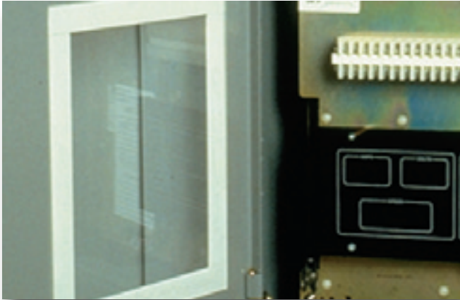
Bond and seal polycarbonate viewing window into the door of a process control system.
