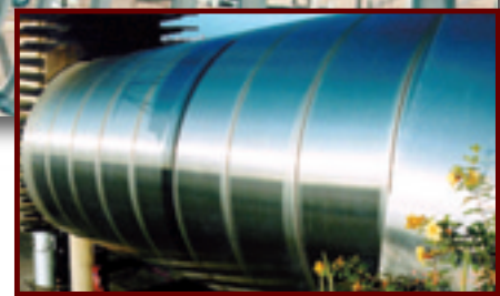
Aeroporto Fortaleza, Fortaleza, Brazil Architect: Claudio Silva, 1997 Stainless steel panels bonded to steel frame.
